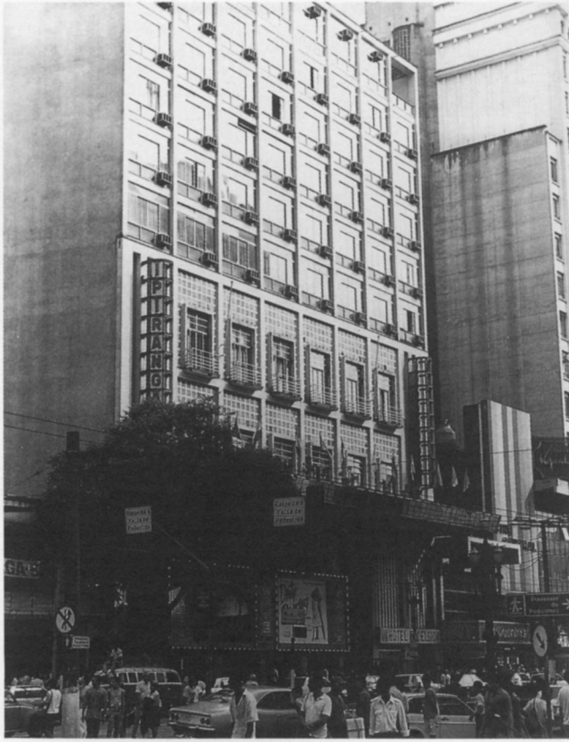
CINE IPIRANGA & HOTEL EXCELSIOR, 1941 Exterior view and detail (the original balcony openings have been filled in with windows); section; and cinema entrance lobby.
